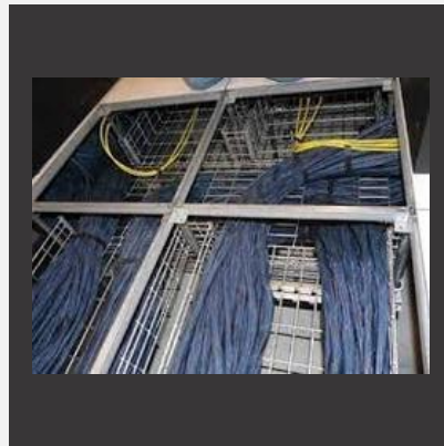
Cabling and Cable Tray Installation
