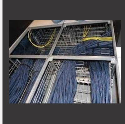
Cabling and Cable Tray Installation
